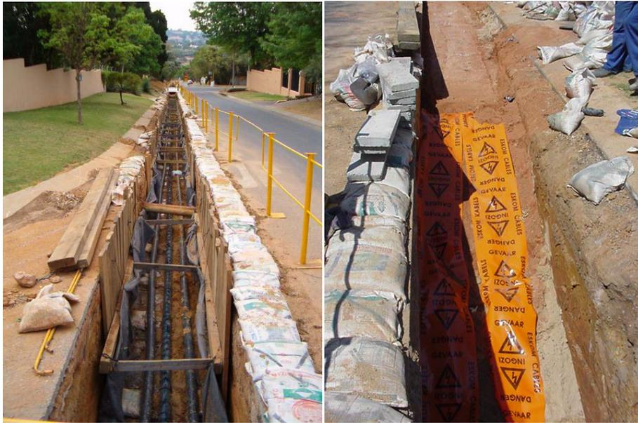
**Figure 2.1: Cable Trenching**
